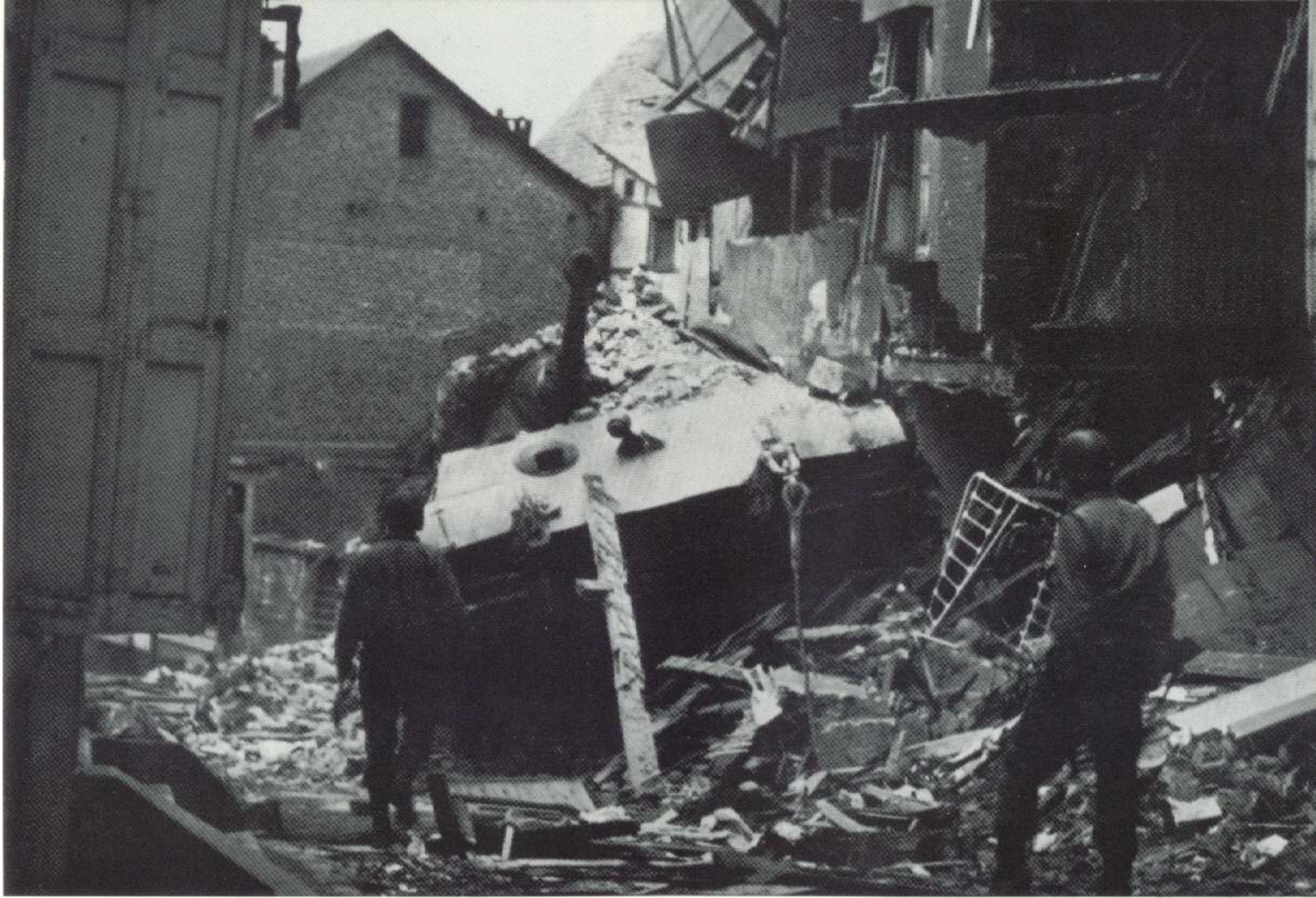
The lead tank of the 1st Company took several frontal hits on the Rue Haute-Rivage in Stavelot and, while moving backward, collided with house No. 9. The tank was stuck in the falling ruins.
